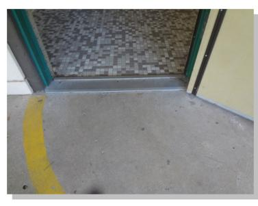
Photo -2 Door thresholds throughout campus have been upgraded to accessibility compliant thresholds
