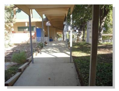
Photo -4 Currently there is no accessible path of travel to building 2, some minor modifications to one of the paths leading to the building will create an accessible pathway
